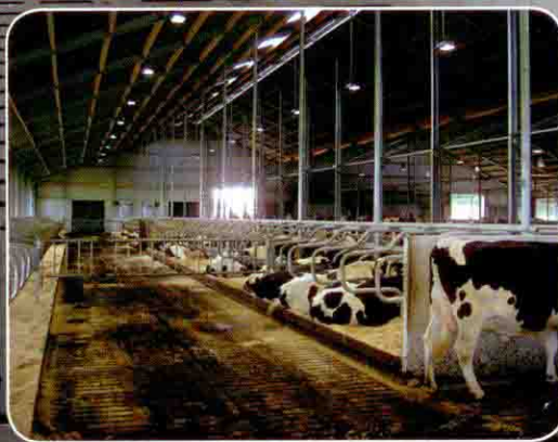
Passageway between two rows at least 2.5 meter
